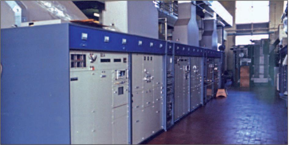
Three 50kW Marconi Doherty transmitters at Droitwich in 1978 for 693kHz (Picture courtesy of John Phillips)
