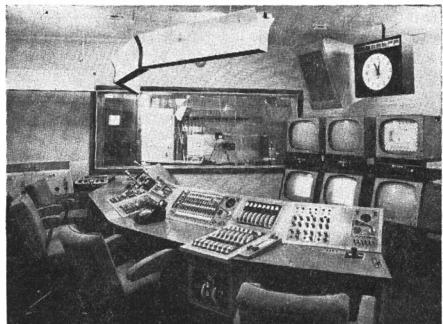
Fig. 6.—Presentation suite: control room and studio.
