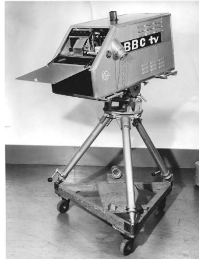
Front cover open to show equipment layout
