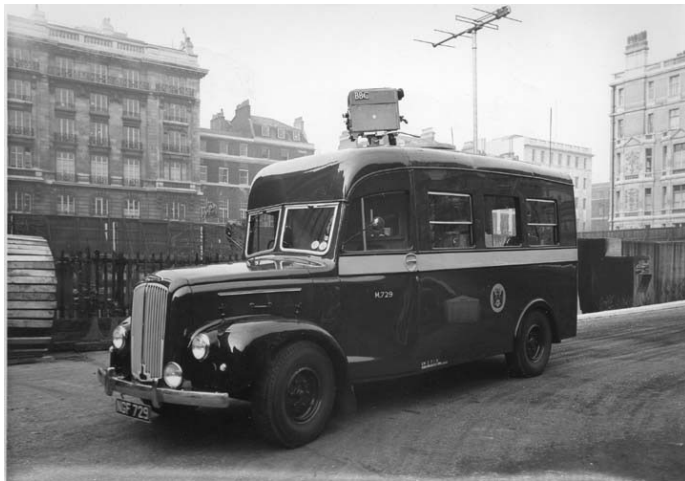
Side view and view showing camera mounting and aerial array.
