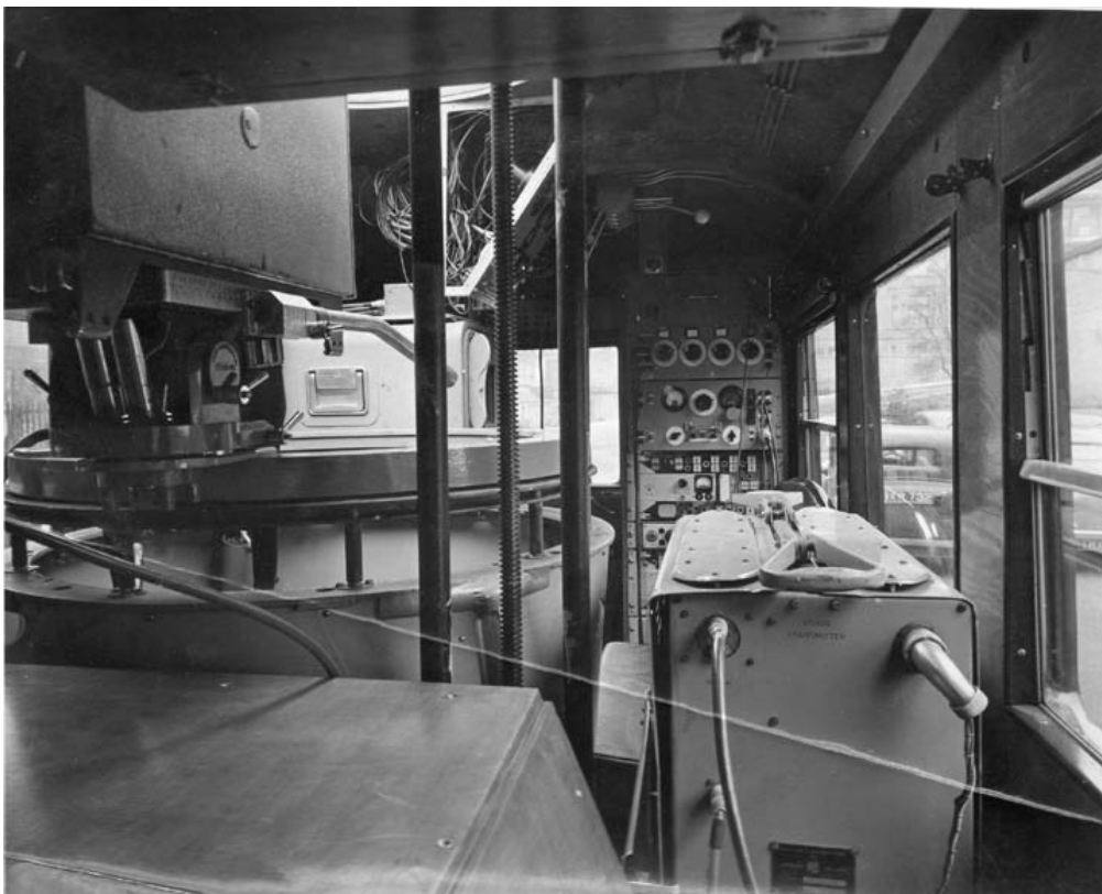
View from the front showing vision transmitter, sound control and communication equipment and camera on lift in down position.
