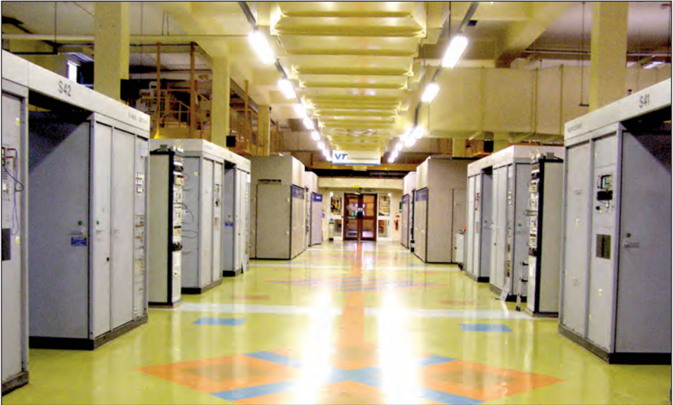
The Sender hall at Rampisham with AEG S4005s in the foreground and Marconi B6127s beyond (Neale Bateman)
