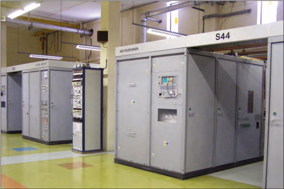
Sender 44 at Rampisham, one of the station's four AEG Telefunken S4005s (Neale Bateman)
