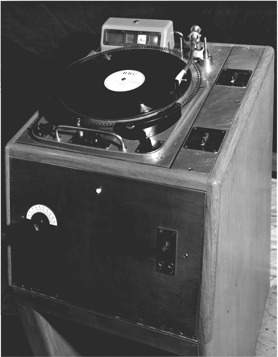
FIG 3 PROTOTYPE MODEL OF FINE GROOVE DISK REPLAY DESK
