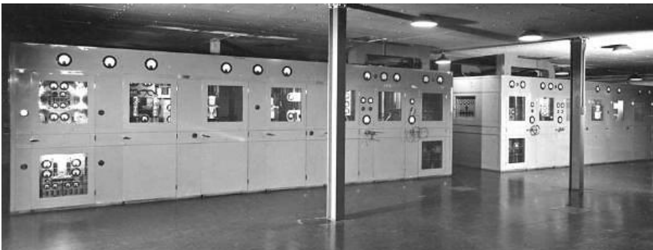
Figure 4. Droitwich 1941. HPMW (OSE6). Two 200 kW Marconi transmitters operating in parallel
