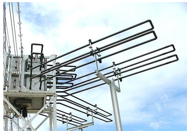
Figure 8. Slew loops for one stack of dipoles on a TCI four-band array. The conductors are just copper 'plumbing pipes' but have the correct diameter and spacing, giving the correct impedance for the signal. Their length gives the correct signal delay for the particular slew bearing required. Photograph courtesy of Pete Bairstow and Babcock Communications
