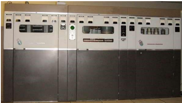
Figure 2. The CE317C 50 kW screen grid-modulated Doherty transmitter as installed at Orfordness. Photograph by Andy Matheson G3ZYP
