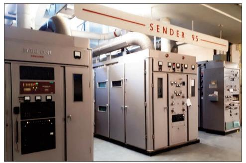
The MWT BD272 at Woofferton showing (L to R) Modulator and Control, RF stages and 5kW driver transmitter (Neale Bateman)
