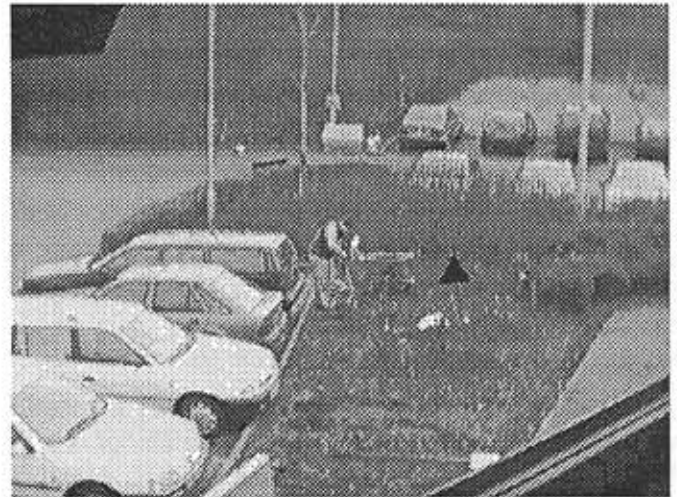
A hole is dug for the first of the parking meters
