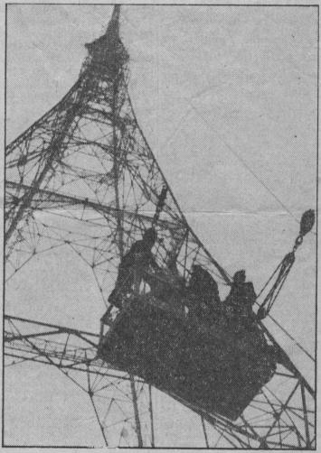
In a cradle, men ascend the B.B.C.'s new 709ft.-high television transmitting tower at Crystal Palace, London, today to fix a dozen rockets to the structure at a height of 625ft. The rockets, each exerting a
