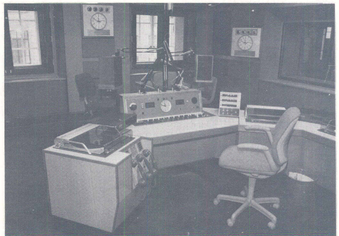
Continuity 3 Cubicle at Bush House
