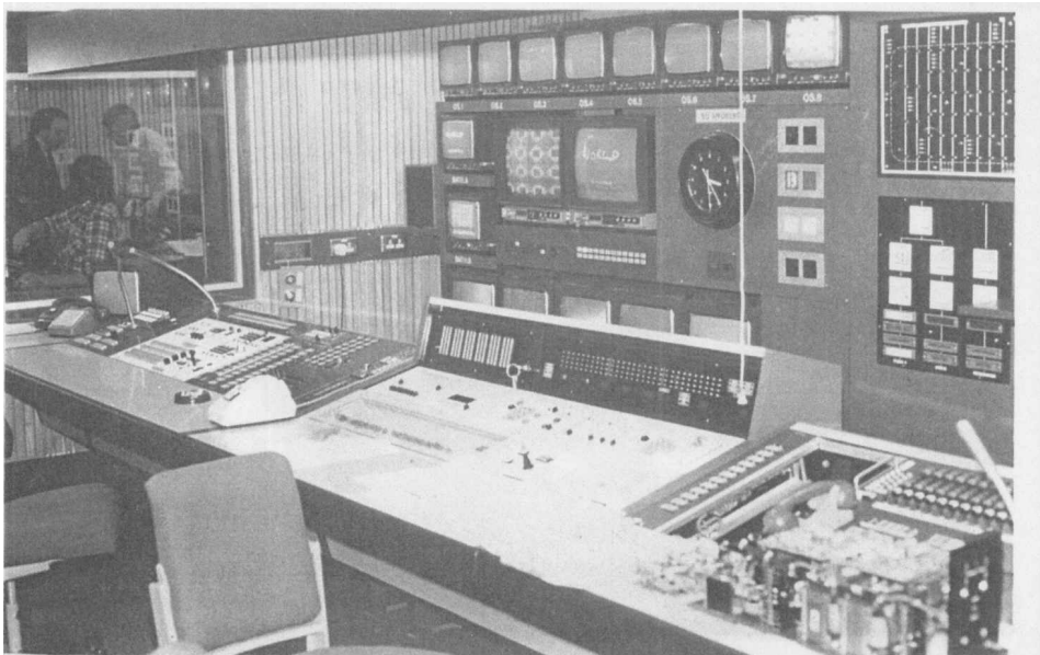
Studio B production and vision control room undergoing acceptance tests
