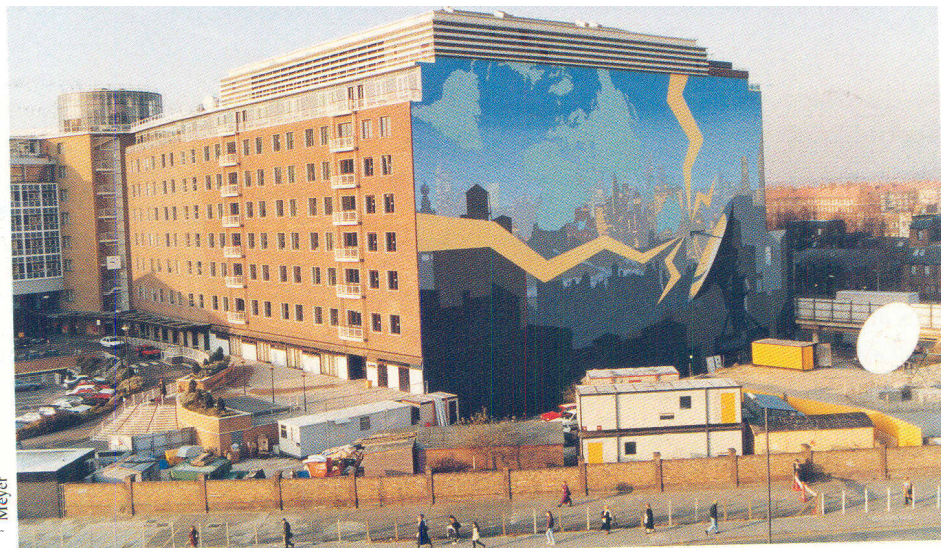
The Stage V extension block at Television Centre showing the mural designed by 15 year old Vicky Askew and, bottom right, the 6m dish antenna referred to on page 20.
