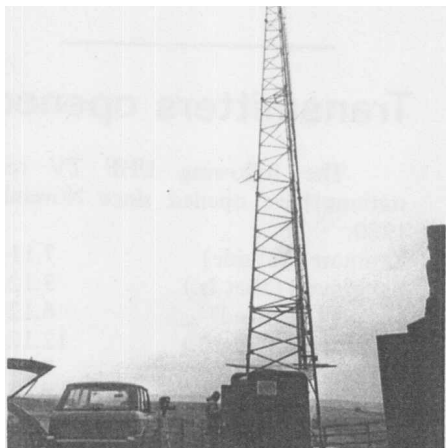
The Hedleyhope mast and transmitter cubicle being filmed as a possible TV news story
