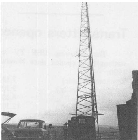
The Hedleyhope mast and transmitter cubicle being filmed as a possible TV news story
