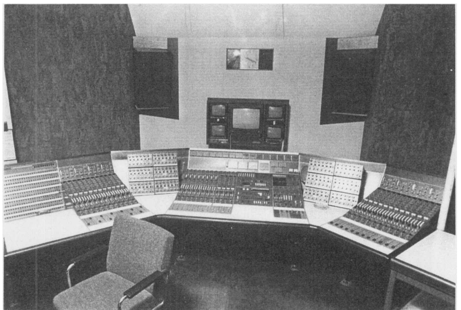
Studio 'C' sound control room
