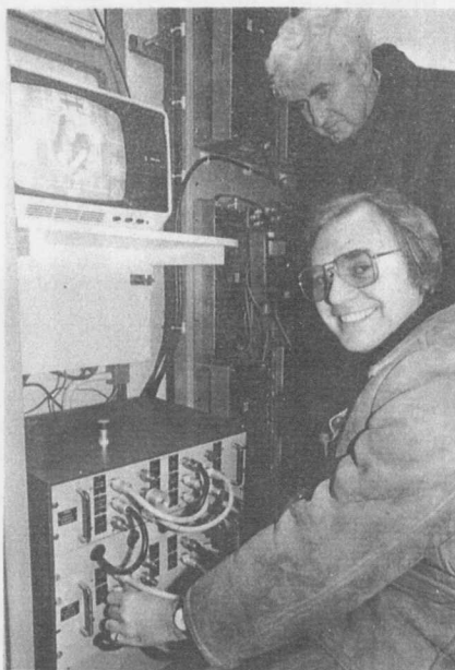
Mike Neville connects the aerial to the transmitters at Hedleyhope, while George MacKenzie makes sure that it is not cross-threaded
